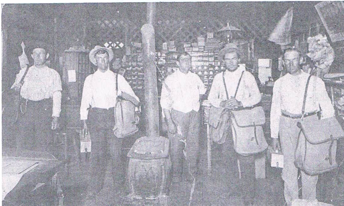
AN EARLY OMAHA POST OFFICE... The Omaha Post Office of this date was on the east side of North Senter Street in a frame building. The lighting was by kerosene lamps and the heat came from a boxed wood stove. Shown left to right: John Clark, carrier; James F. Hill, carrier; W. W. McCollum, Postmaster; J. E. (Erb) Davis, carrier; W. C. (Will) Allen, carrier. Mr. McCollum served under the McKinley, Roosevelt and Taft presidential administrations. Photo courtesy of Joe E. Hill, 2914 Marx, San Angelo, Texas.
